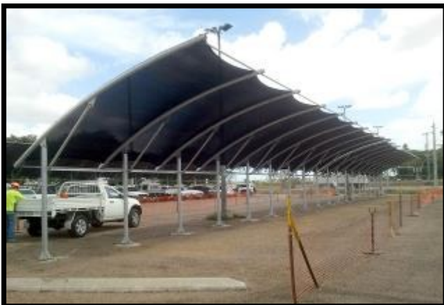
CAR PARK SHADE STRUCTURE WILMAR SUGAR — BRANDON MILL
